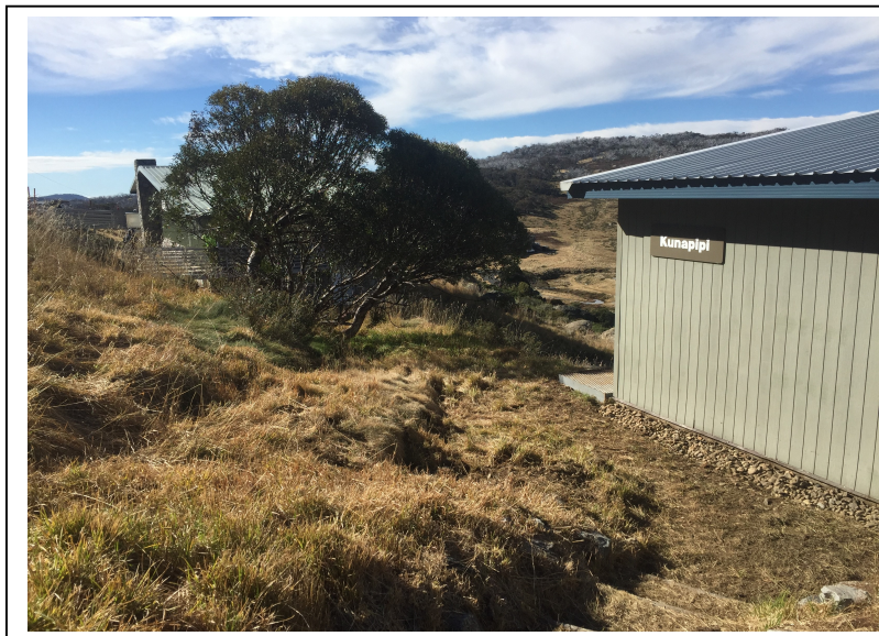
Evidence of remaining benches from access road construction to Yalara Ski Lodge. Yalara is the building behind the Snow Gum, proposed steps and deck are in front of this gum on disturbed land. Photo 2018
