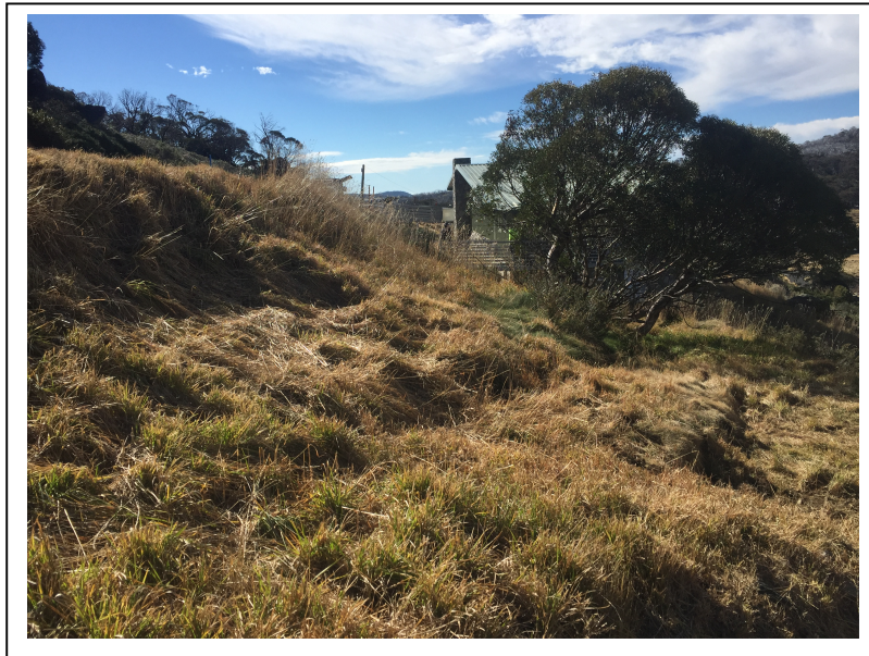
Evidence of remaining benches from access road construction to Yalara Ski Lodge. Yalara is the building behind the Snow Gum, proposed steps and deck are in front of this gum on disturbed land. Photo 2018.
